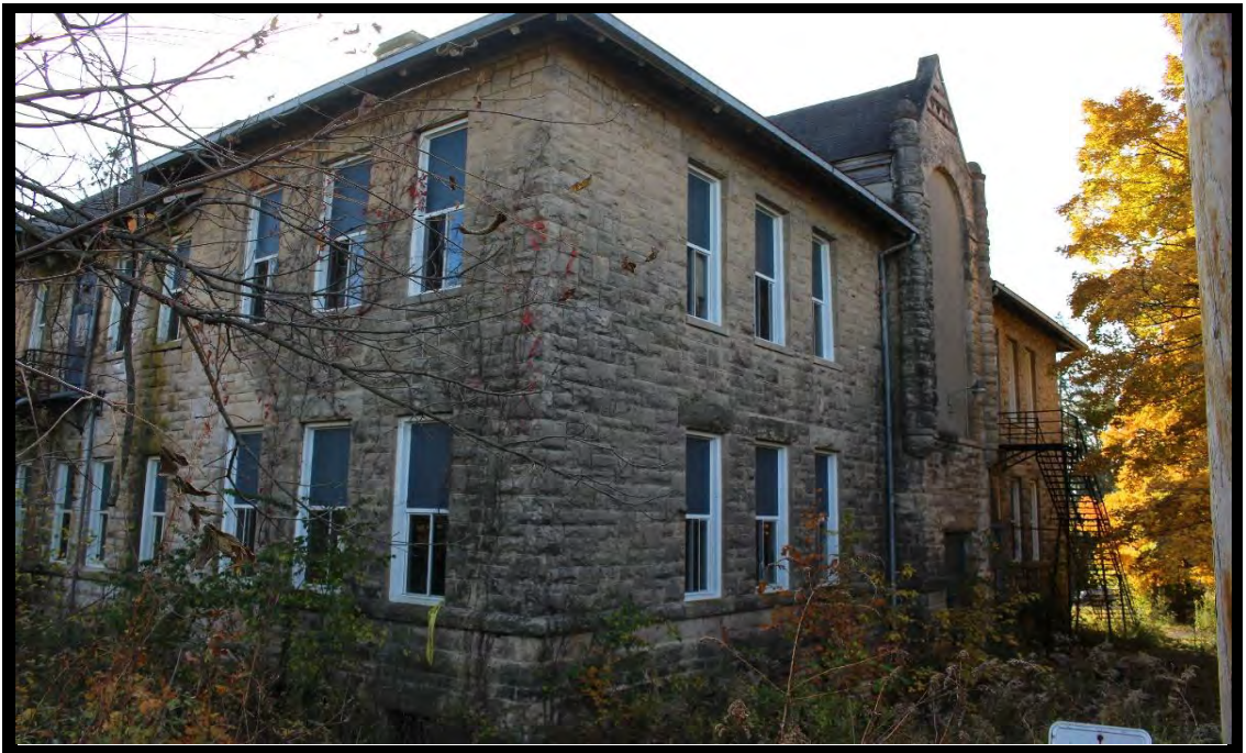
4 The northwest corner of the building.
