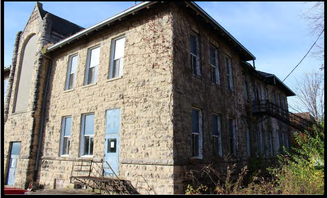
3 The northeast corner of the building.
