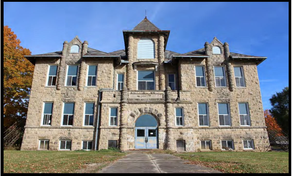
1 420 West Columbus Street, West Liberty, Ohio is the site of a former school building, which was built in 1916. The south side of the building.
